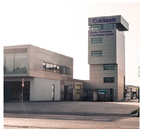
Hydro-Dynamics Experience Centre in Netherlands
